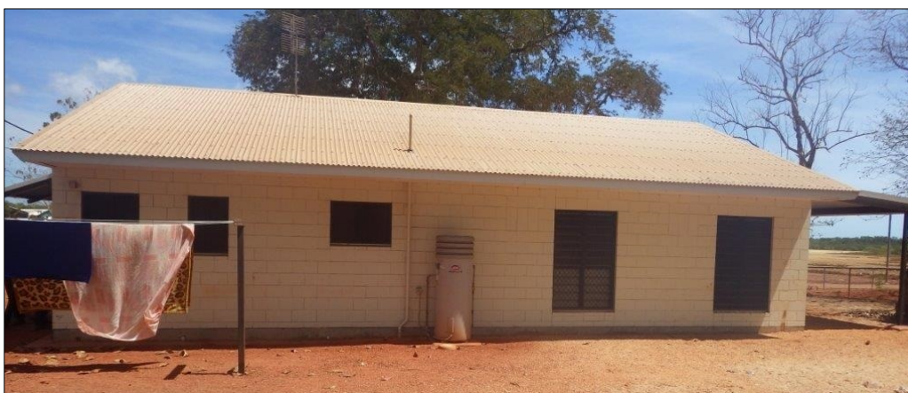
Typical new three-bedroom house, with core-filled concrete block walls and heat pump hot water system.
