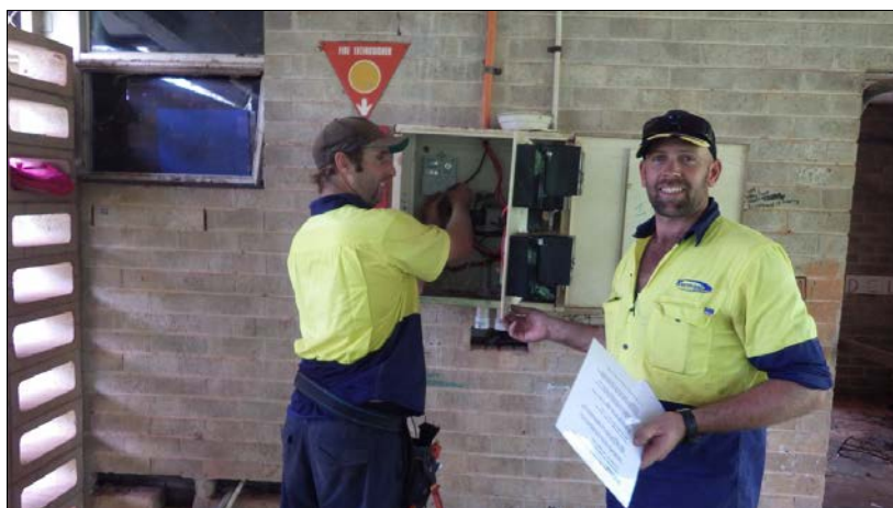
Contractors installing data loggers
