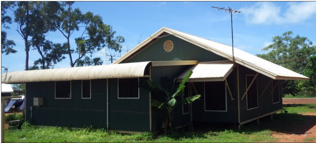
Lightweight construction raised floor: refurbished.
