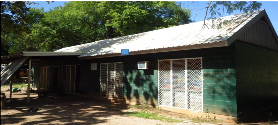
Refurbished concrete block slab-on-ground three-bedroom housing – three examples.
