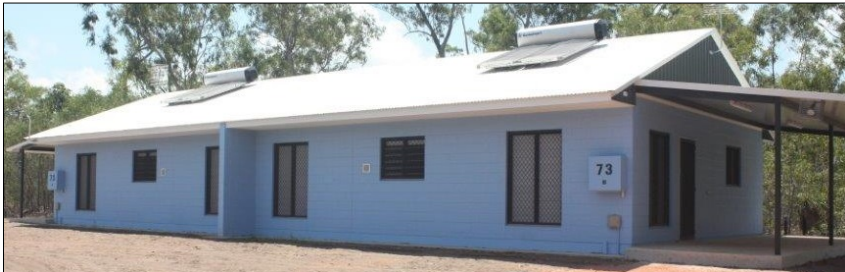
Typical duplex, new housing style with two bedrooms per unit, core-filled concrete block walls and concrete slab, Bondor insulated panel ceiling.
