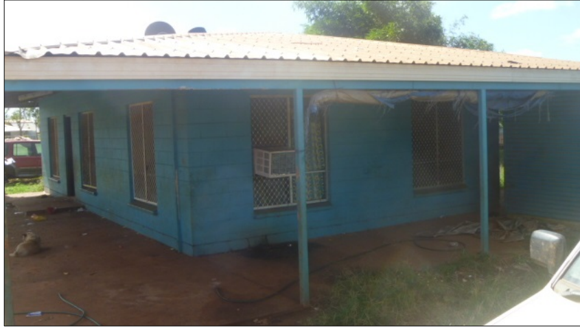
Four-bedroom concrete block slab-on-ground refurbished house.
