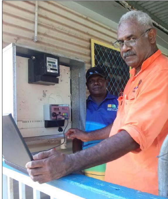
YEEW assisting a contractor in Galiwin'ku to install a BEEBox
