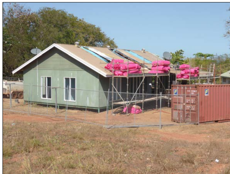
Ceiling insulation being installed in Yirrkala
